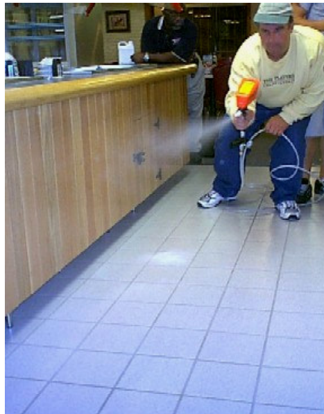
Application in progress
